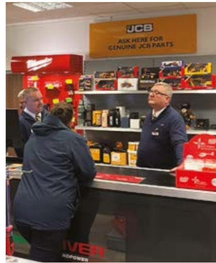
First tasks included installing a new parts counter and storage, fitting out office space, and installing an integral bulk oil system
