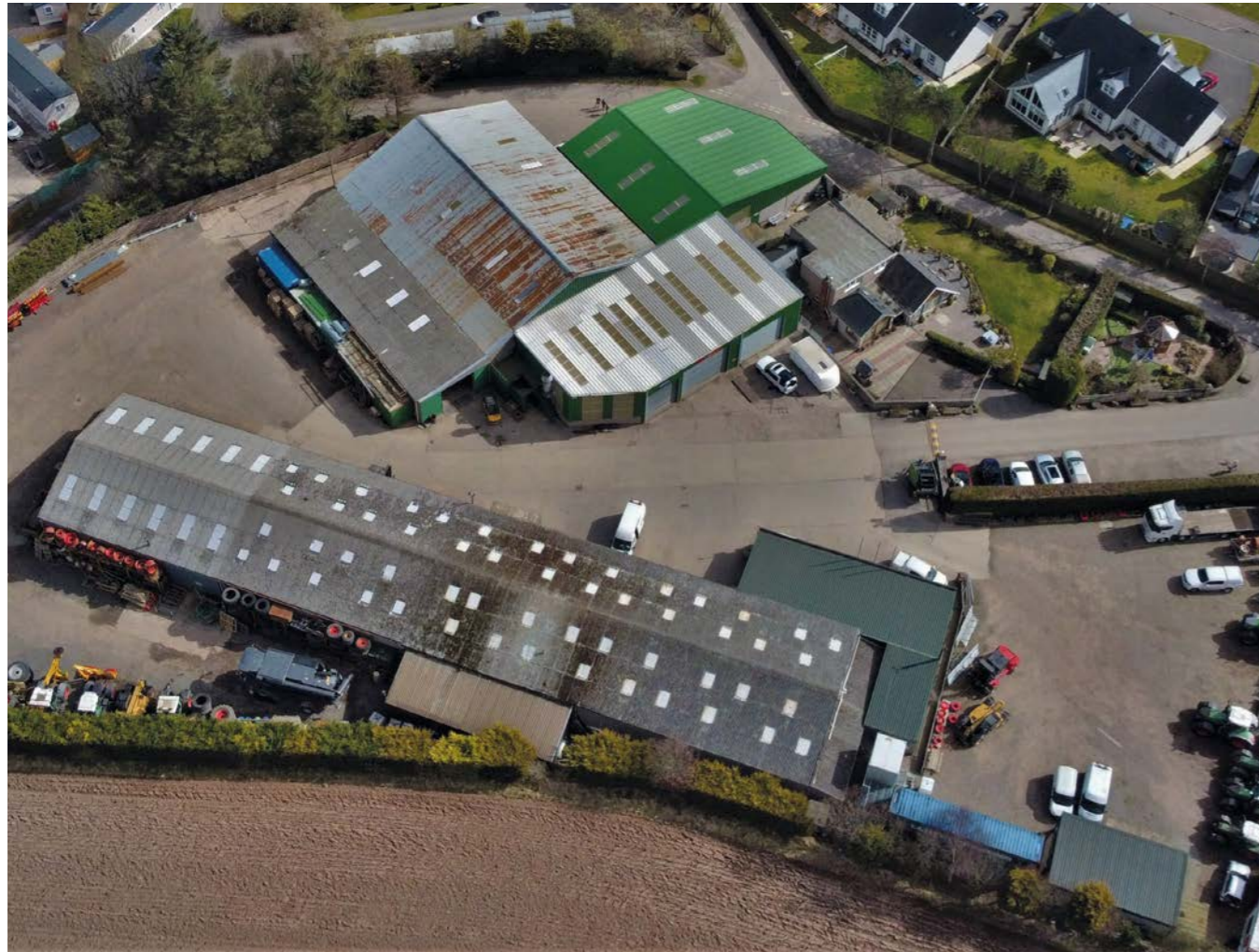
Recent investments in infrastructure have included new workshops, built in 2017, at the St Cyrus main depot
