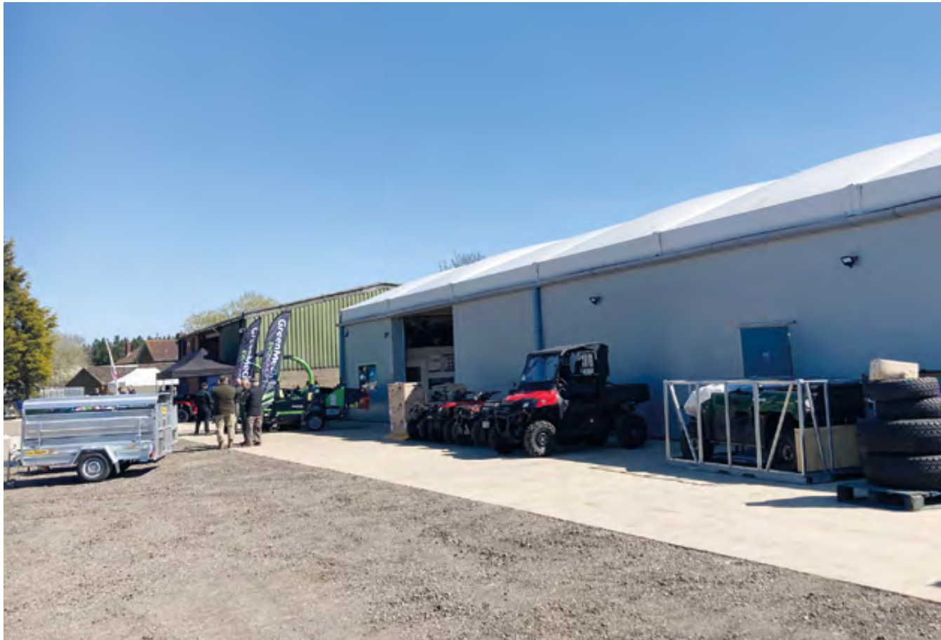
A 10 x 30m semi-permanent building is currently providing workshop facilities, and will be turned over to storage once the new 50 x 20m permanent building is constructed
