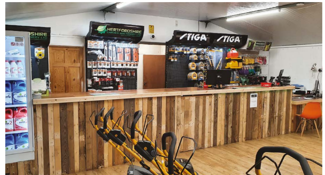
“The new counter constructed from reused crates and pallets, with a countertop made of repurposed wood flooring”
